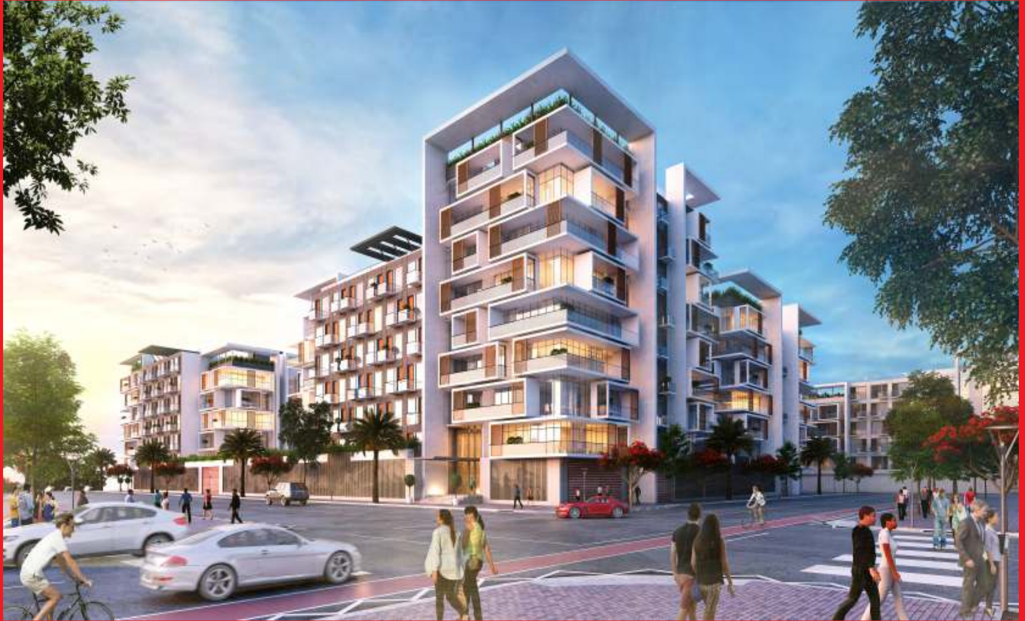
Victoria, Proposed Residential Developments at Meydan, Dubai. | Client : M/s. Azizi Developments LLC
