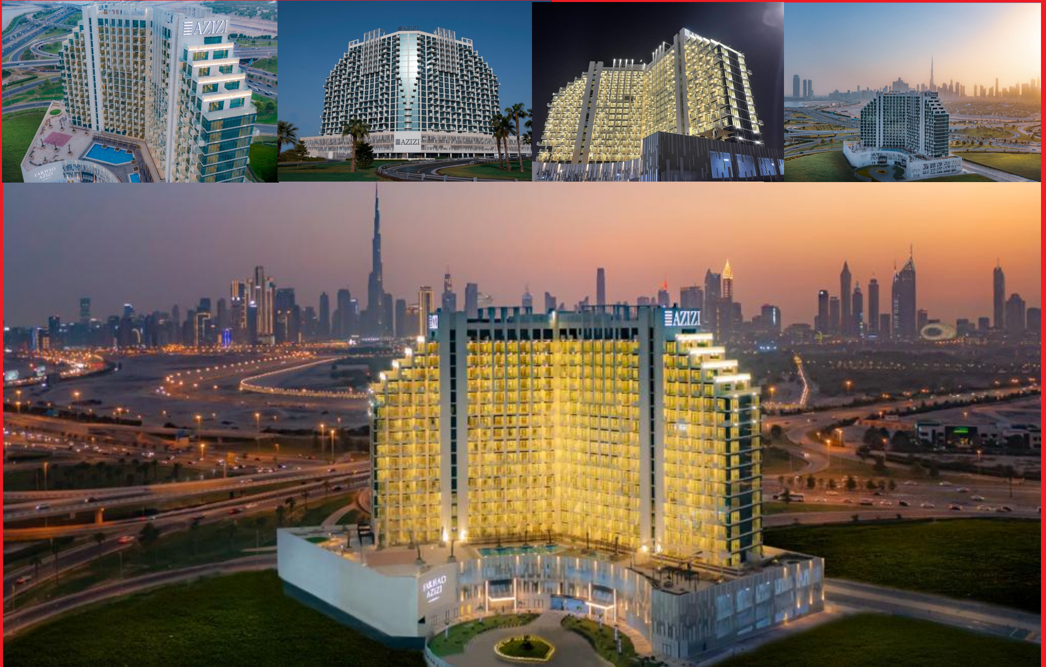
(B+G+2P+17 Typ floor) Residential Building at Dubai Health Care City Phase-II, Dubai. | Client : M/s. Azizi Developments LLC
