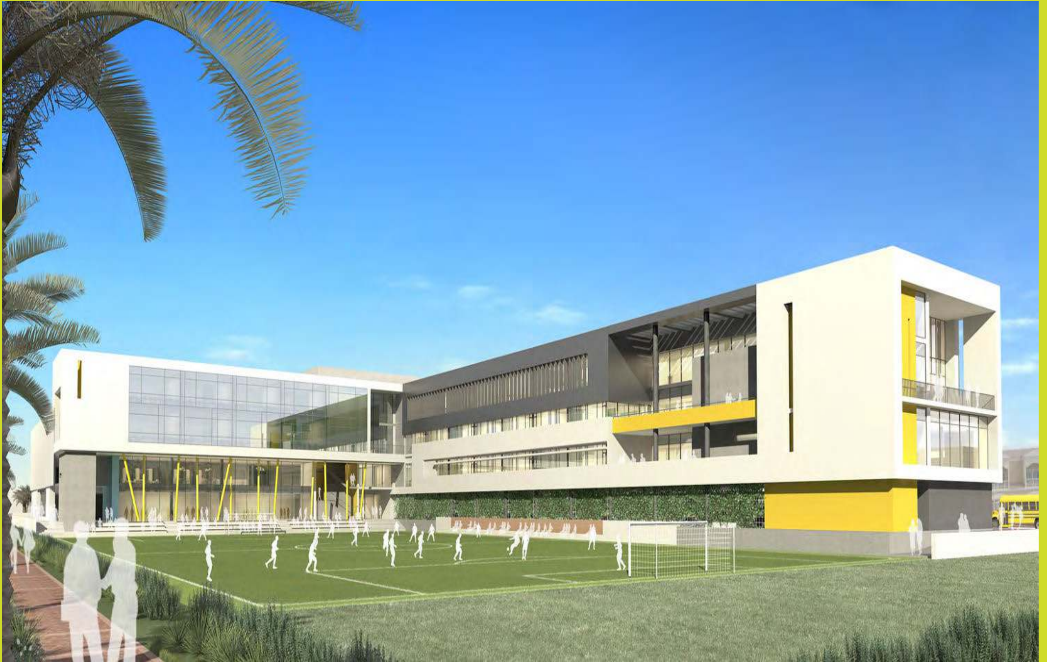
(B+G+3) Arcadia Secondary School, JVT, Dubai | Client: M/s. Global Oasis Properties LLC & Arcadia Investment LTD
