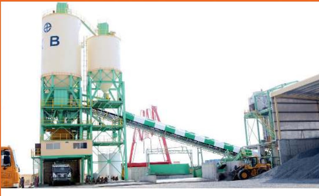
Concrete Batching Plant, Ajman | Client : M/s. K B Remicon, Head Office, South Korea
