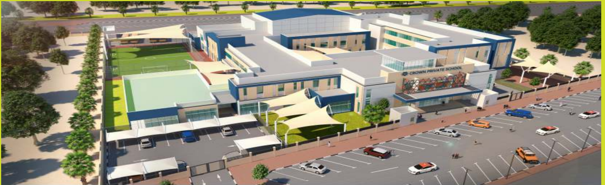
G+2 Crown Private School, Ajman | Client: M/s. Ajman Properties Corporation (AQAAR)
