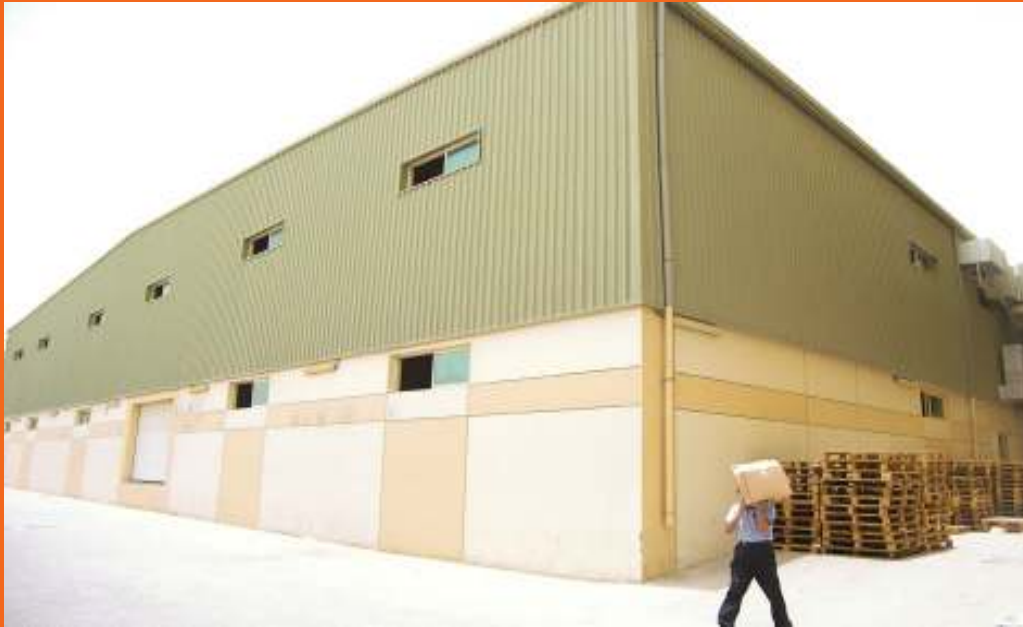
Medicine & Cosmetic Store - Industrial Warehouse, Ajman | Client : M/s. New Medical Centre (NMC), UAE
